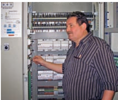
Reinhold Buschle adjusts the \dot{V}_{MIN} and \dot{V}_{MAX} parameters of the VAV controllers on the Fan Optimiser.
