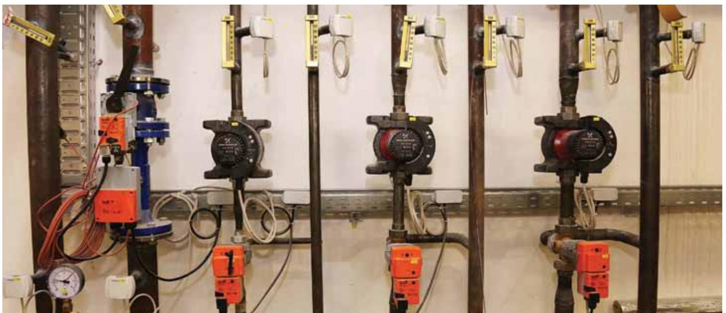
On left in photo of return pipe: one of the eight Belimo Energy Valves™ installed in the Ludmillenstift heating circuit
